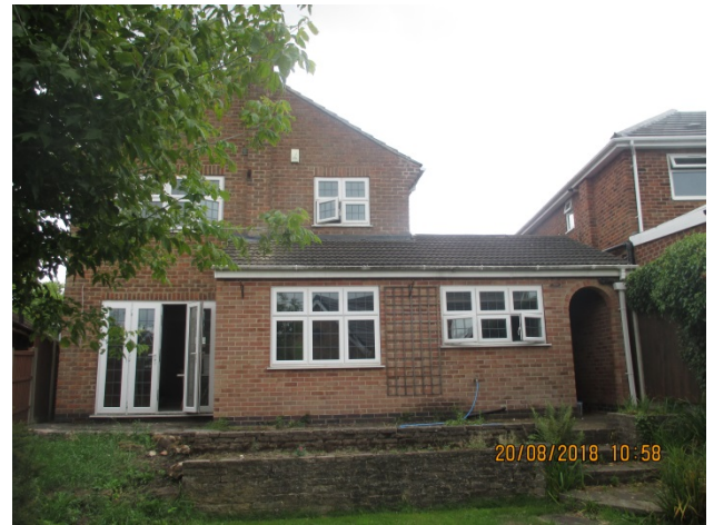
View of north west (rear) elevation
